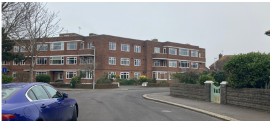
Figure 35: Low brick boundary walls around Winchelsea Gardens
