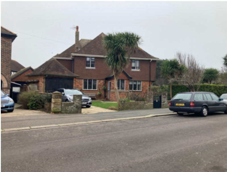
Figure 29: No.2 Dover Road
