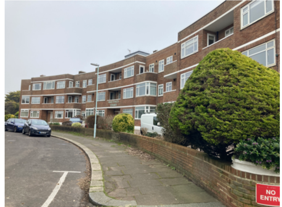
Figure 26: Hastings Court front elevation
