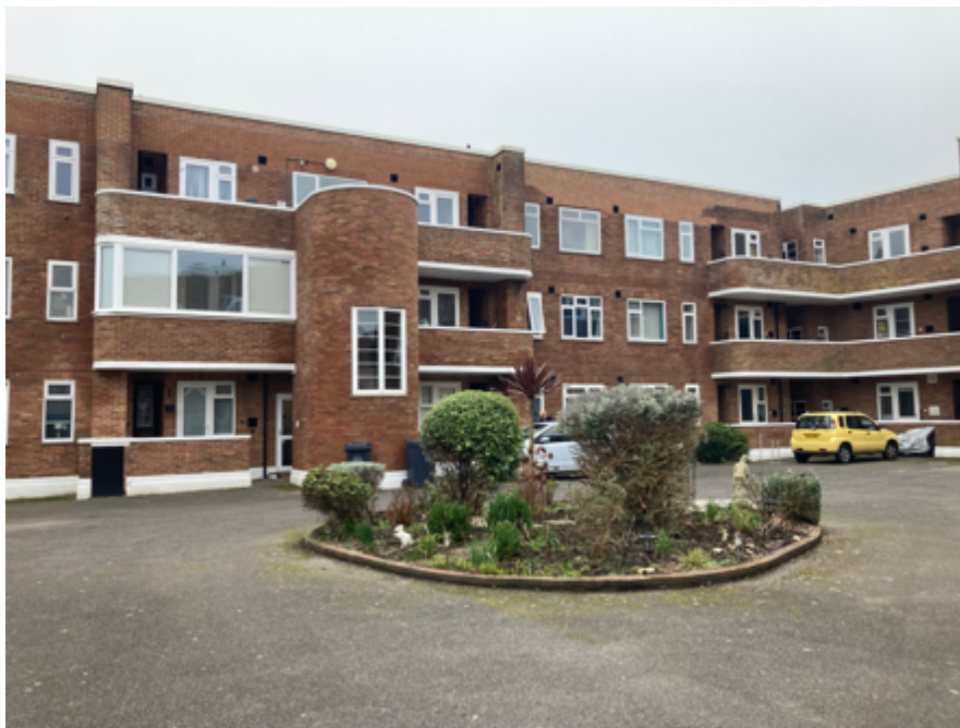
Figure 27: Winchelsea Court, rear elevation
